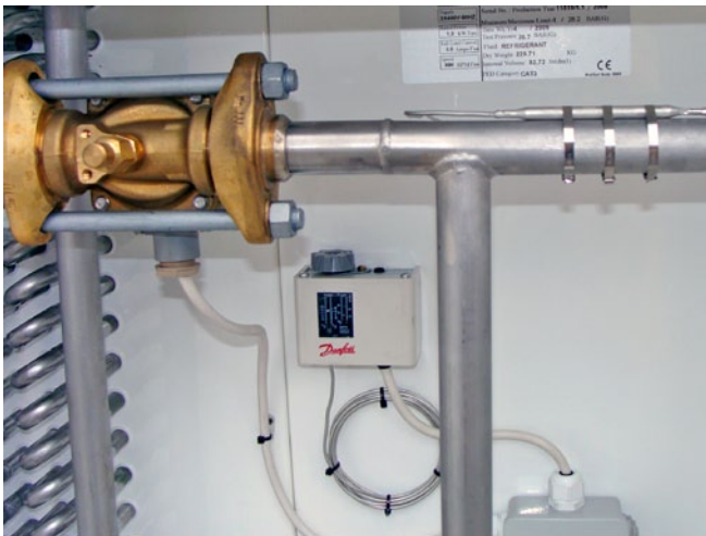
1'000 kg/hr Atmospheric CO 2 Vaporiser Thermostat
